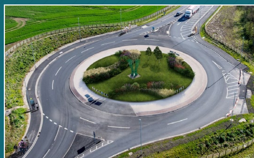
New A635 access roundabout
